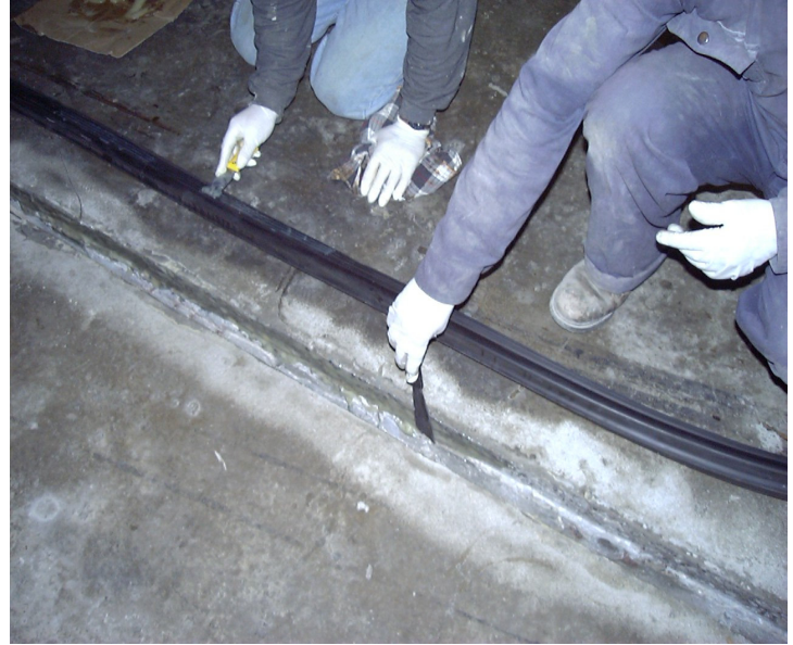
Application of adhesive to joint surface.
