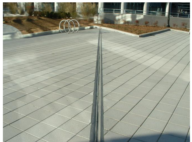
Completed plaza deck with expansion joints installed
