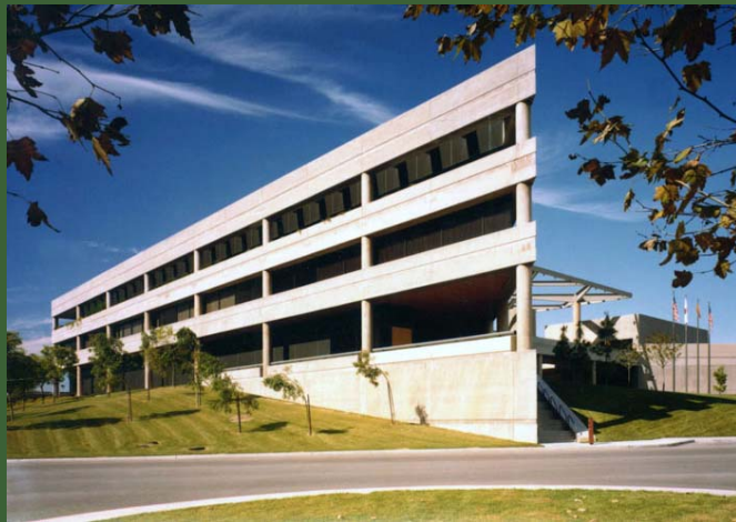
Brea Civic Center Brea, CA
