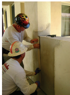
Color-matched expanding foam seal blends in well with its surroundings
