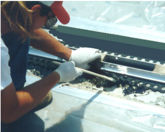
Installation of CR-Series expansion joint
